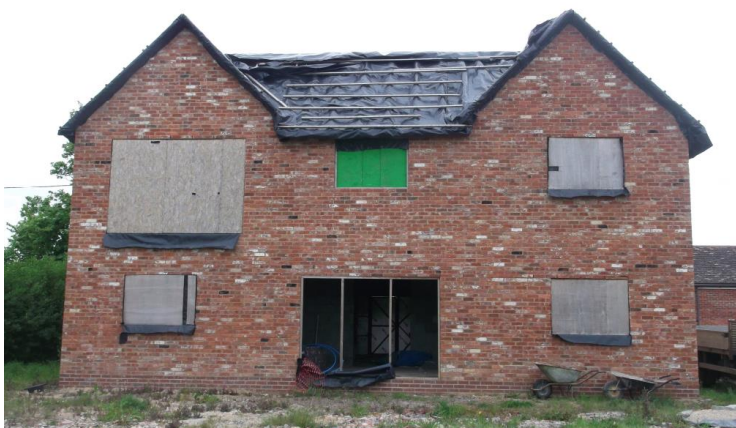
Photo of unauthorised dwelling on site
